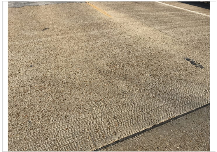
Longitudinal cracks and abrasion
