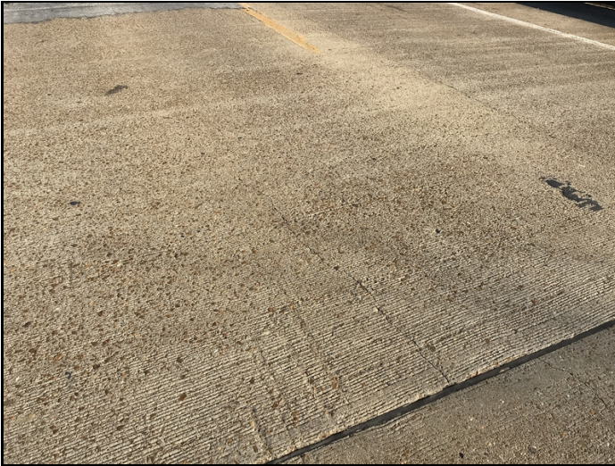
Longitudinal cracks and abrasion
