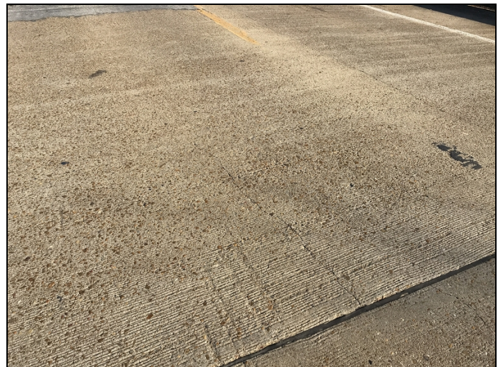
Longitudinal cracks and abrasion
